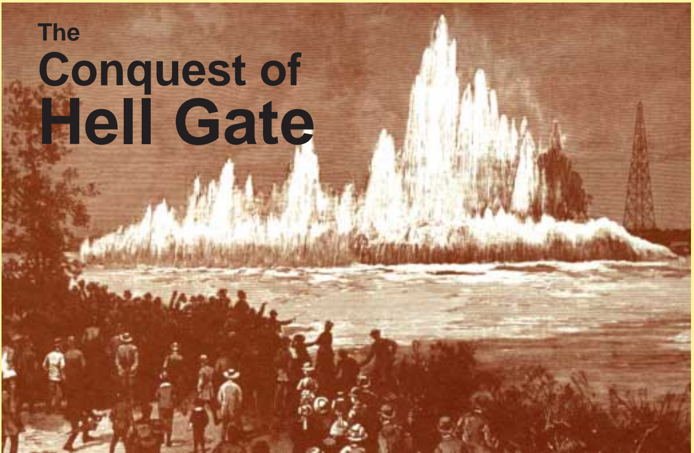
The Great Blast of Flood Rock in 1885 “The greatest quantity of explosives ever attempted in a single operation.” Fifty-thousand people crowded both shores of the East River to witness the great underwater explosion that leveled the rocky reef which made navigating Hell Gate very hazardous.
